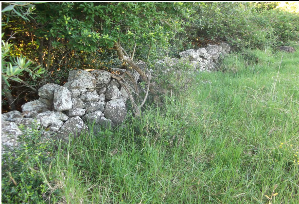
Photo 3: View of stone fence along the eastern boundary
